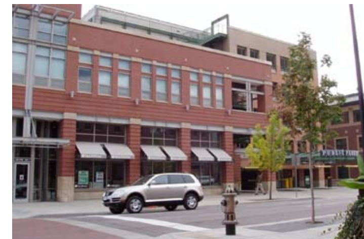
Parking structures that blend into urban form and offer ground floor retail
